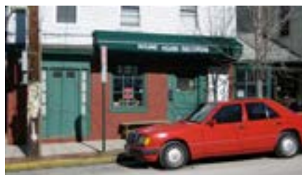
The blank walls and windows are uninteresting and shoppers may pass on by.
