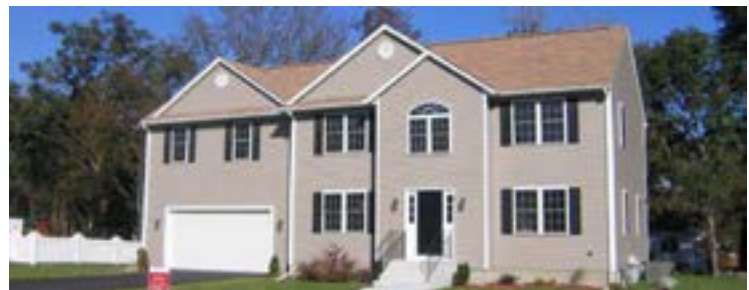
This building has been overly complicated by too many roof forms. The additional ridges, valleys and eaves are a maintenance liability.
