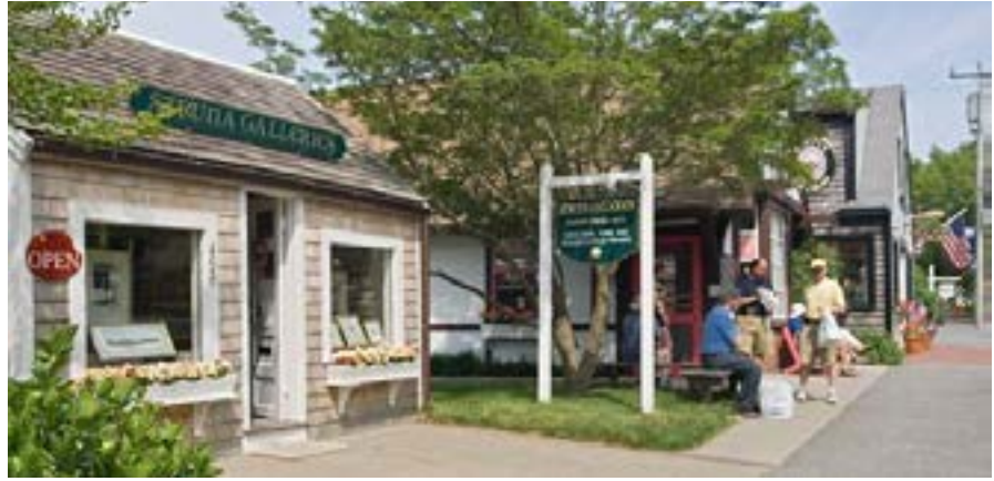
Buildings in a village have varying setbacks but still relate to the street.
