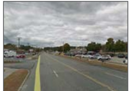
Deep setbacks, endless parking lots, and frequent curb cuts make walking along Route 1 unpleasant and dangerous
