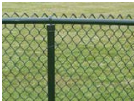
Chain-link fencing should be confined to the least visible locations.
